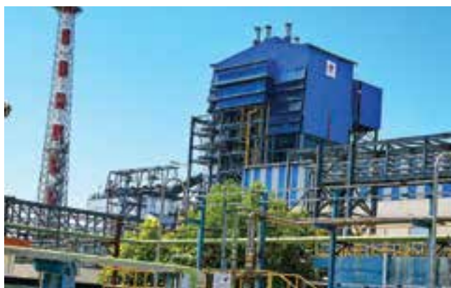
▲ CFBC Boiler Facility at Dahej.
