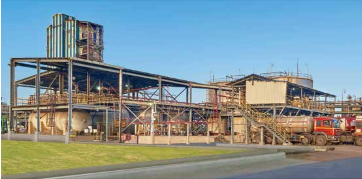
▲ Nitric Acid storage and despatch section at Dahej.
