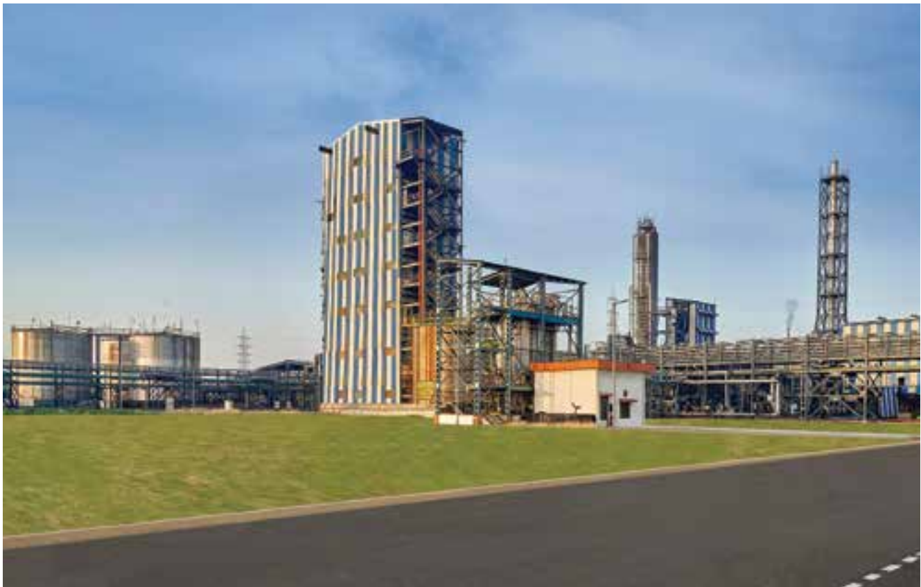
▲ Concentrated Nitric Acid Plant at Dahej.
